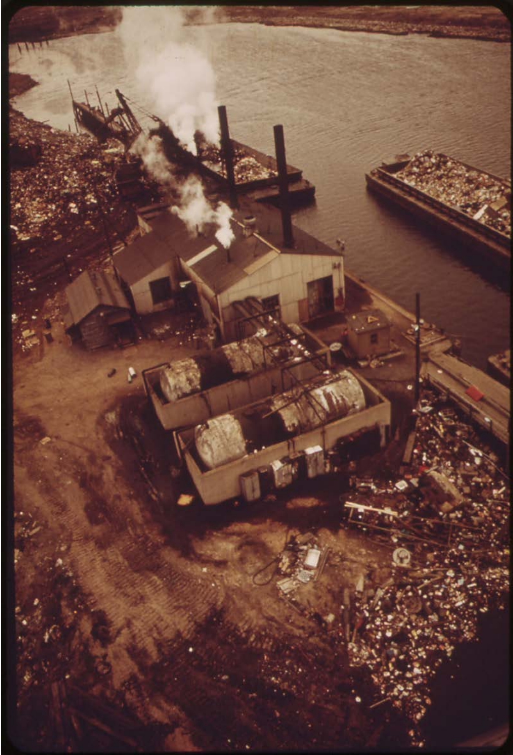
Figure 28. Docks at Fresh Kills Landfill. Source: U.S. National Archives; Public Domain. This image, from 1973, shows the transfer station and cranes at the docks of Fresh Kills.
