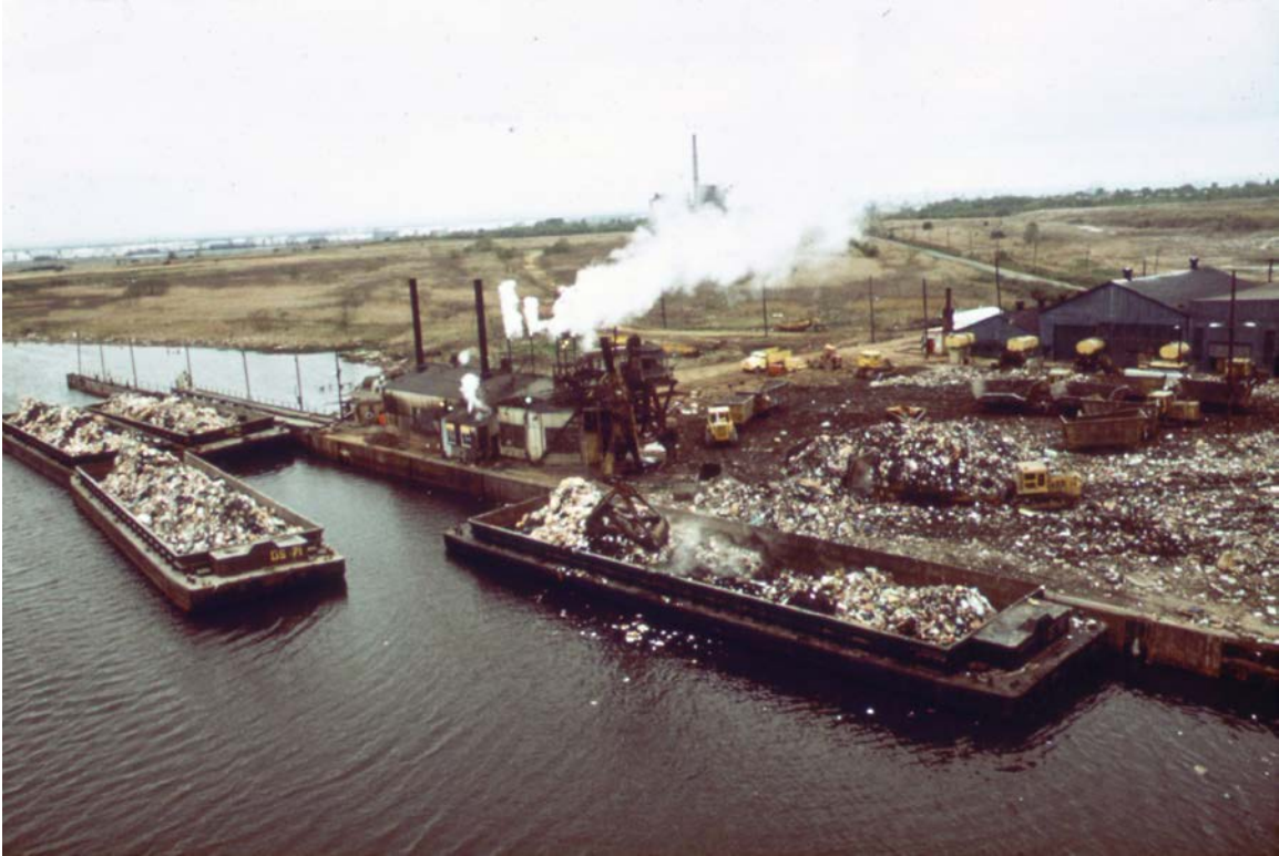
Figure 27. Garbage Scows Unloading at Fresh Kills. Source: U.S. National Archives; Public Domain. Garbage Barges were the primary means of shipping garbage from New York's boroughs out to Fresh Kills. This picture, from 1973, illustrates the process of transferring garbage from barges unto trucks upon arrival at the landfill.
